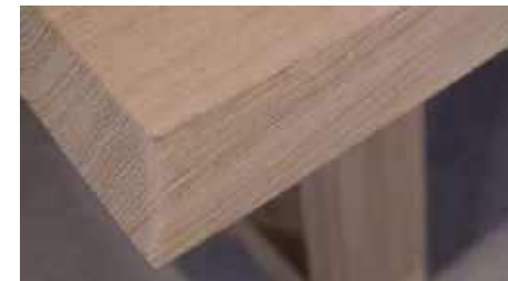
Edges beveled outwards on all sides
